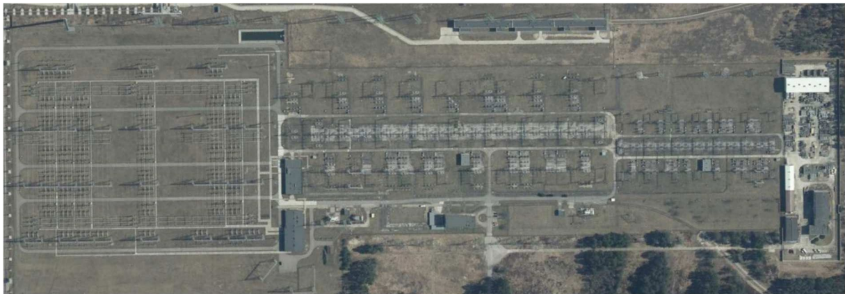
Figure 23 Koźienice Power Station
